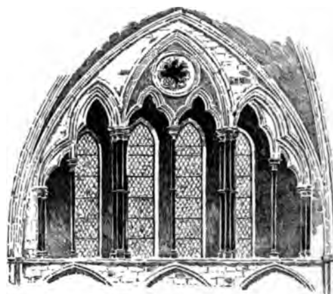
INTERIOR OF CLEARSTORY-WINDOW, NORTH ARM OF TRANSEPT.
